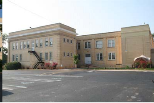
Pound Hall, side facade
